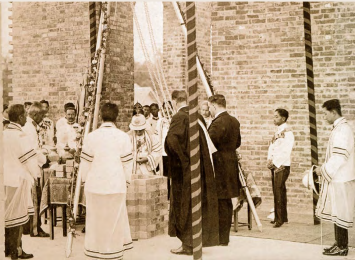
King Vajiravudh laying the foundation stone of the Headquarters of the Civil Service College of King Chulalongkorn on January 3, 1915, which is now Maha Chulalongkorn Building, Chulalongkorn University.
