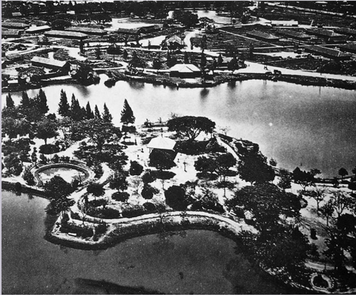
Lumphini during construction
