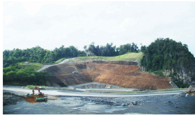
Quarry site at Thung Song cement plant in 2010
