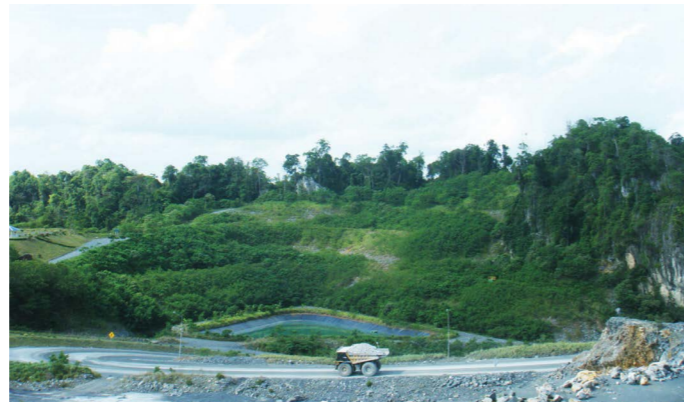
Quarry site at Thung Song cement plant in 2012
